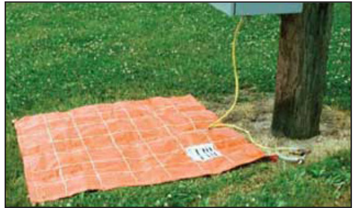
Overhead Distribution and Transmission Switches
